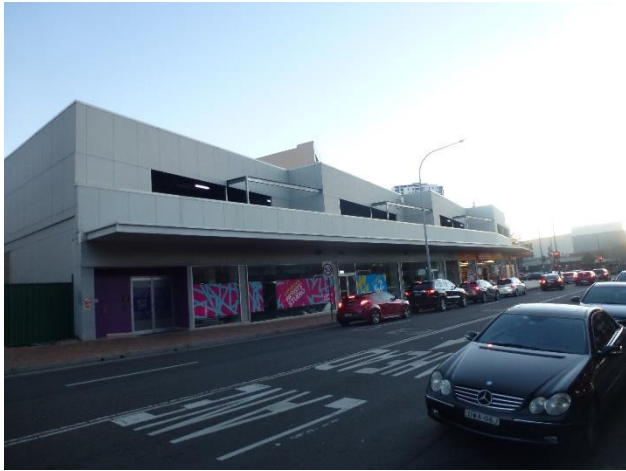
Figure 2-3 Commercial building occupying the site as viewed from Scott Street (north east)
