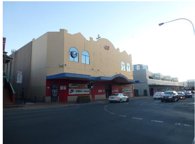
Figure 2-6 Commercial building occupying the site as viewed from Scott Street (north east)
