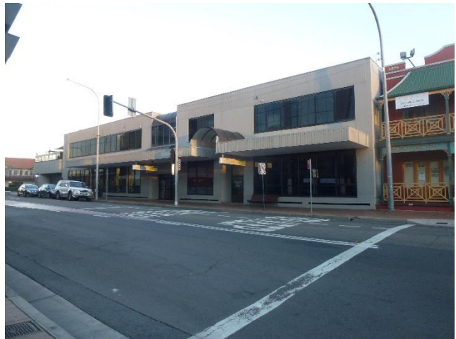
Figure 2-15 Two storey commercial building at the intersection of Scott and Terminus Street
