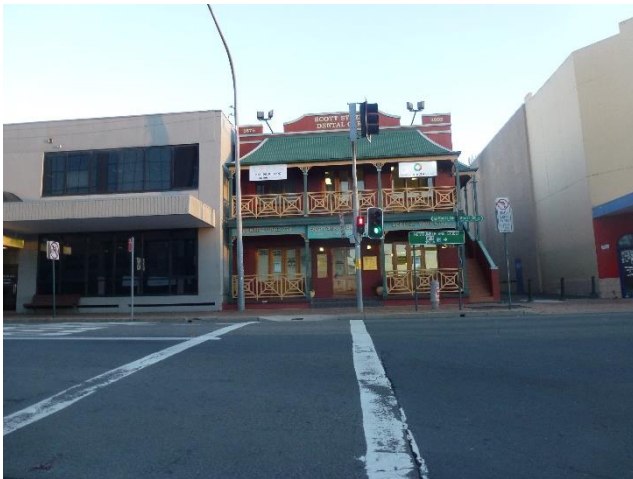
Figure 2-14 Two storey commercial building to the east of the George Street through site link
