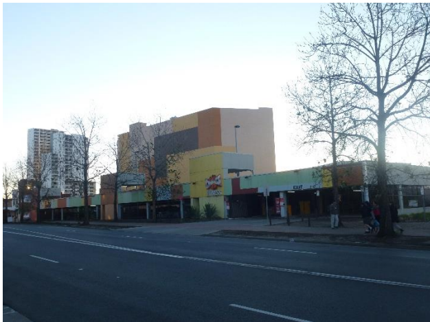
Figure 2-5 Above ground car parking structure as viewed from Terminus Street (south east)
